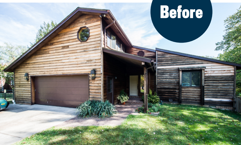
Original Redwood Siding in deteriorated condition
